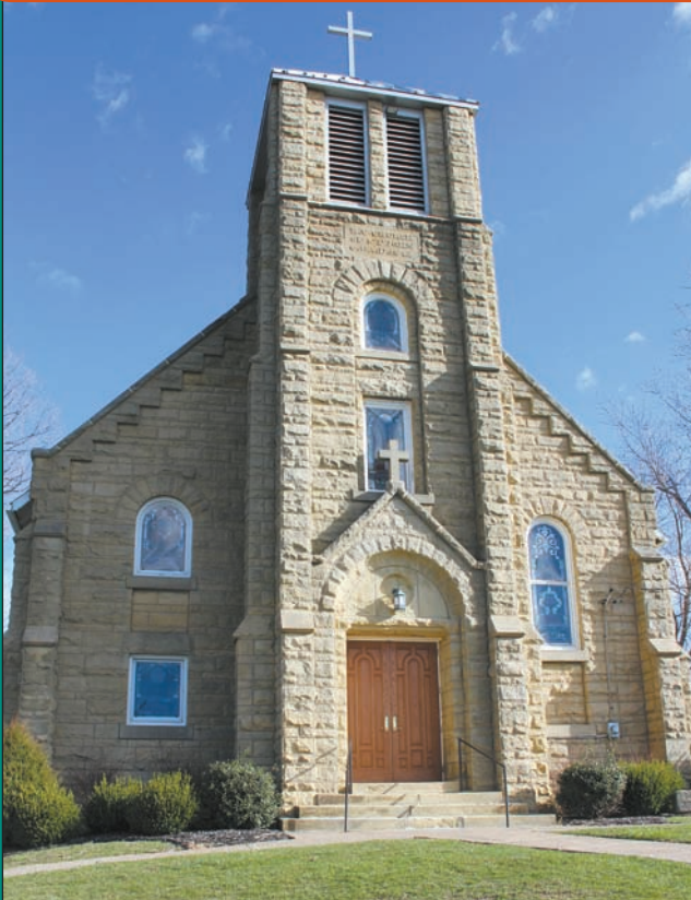
repointing the stone on St. John the Baptist Church, Miltonsburg, said Father David L. Gaydosik, pastor;
