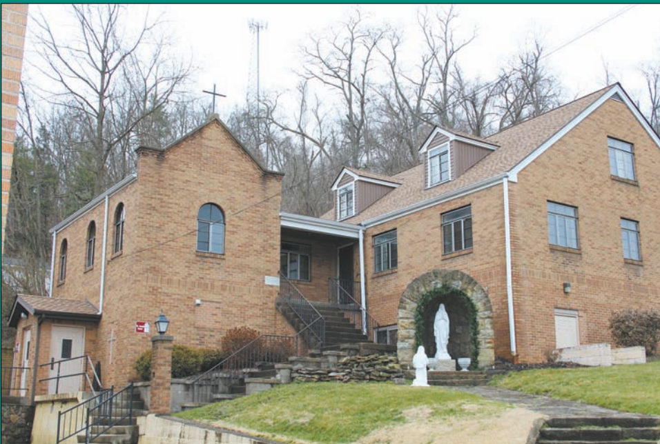
replacing the roof on the former convent at St. Joseph Church, Bridgeport, that now serves St. Joseph parishioners as their parish center, said Father John F. Mucha, pastor; and
