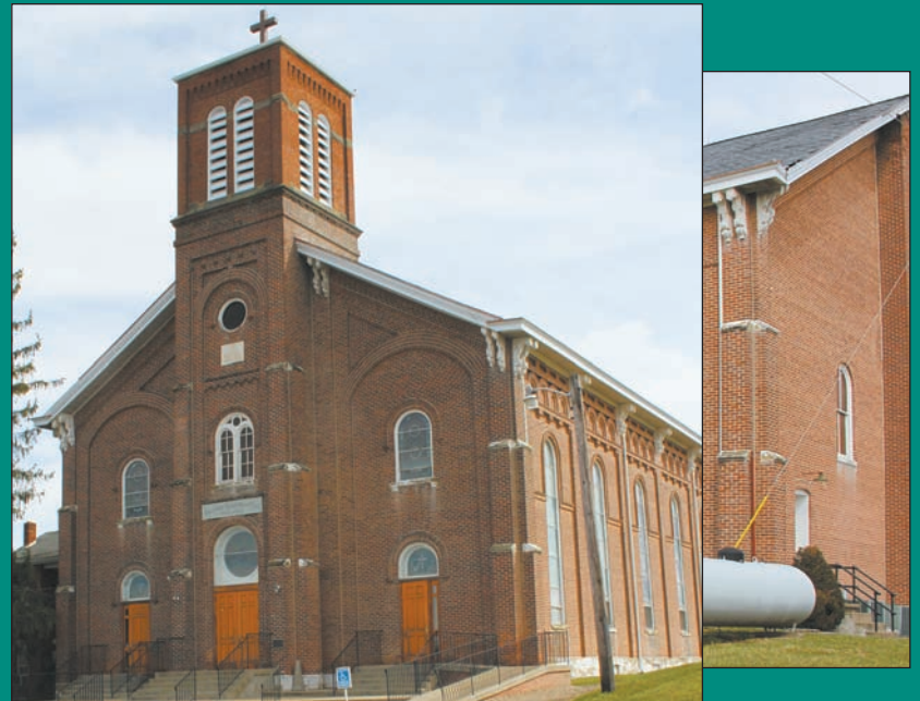
maintaining St. Mary of the Immaculate Conception Church, Fulda, that was built in 1875, and where work continues on the outside, said Father Wayne E. Morris, pastor.
